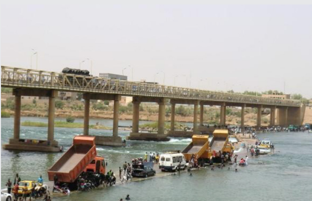
Road way on river
