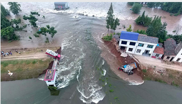
Gap of a broken dike in Huarong county
