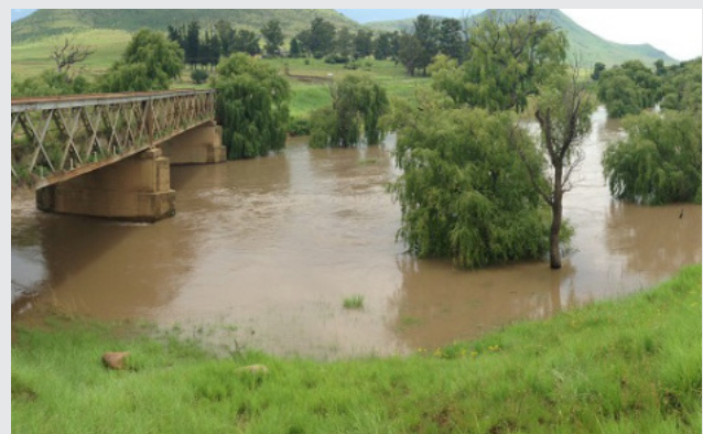
Bridge over uMzimvubu Catchment
