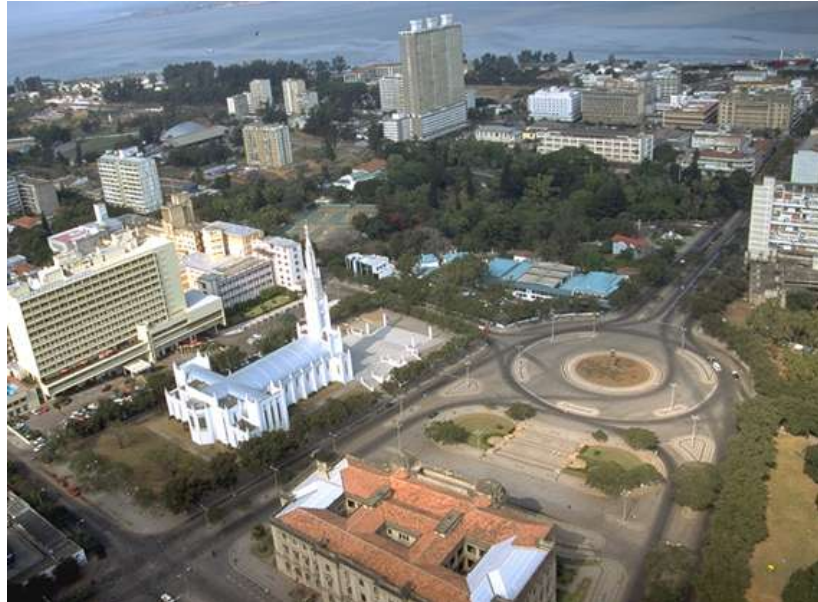
Figure 6. The 'cement city' or centre of Maputo City 8 .
