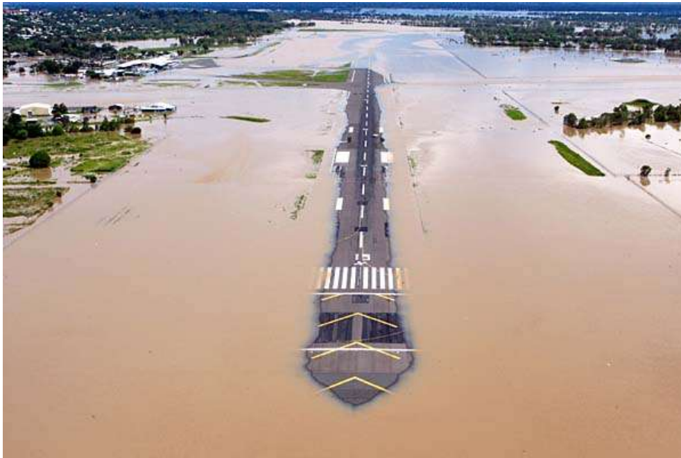
Figure 12. A flooded runway in Rockhampton, Australia leaves boats as the only viable transport until the flood water subsides. 15
