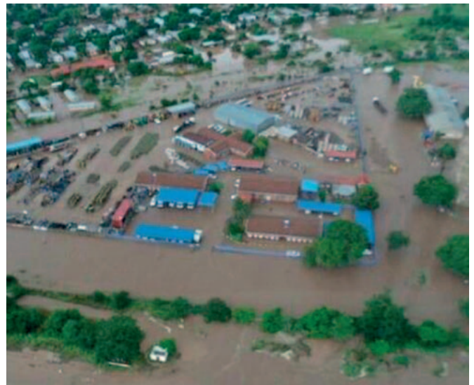
FIGURE 21: Flooding in Bela-Bela causing extensive infrastructure damage. 31
