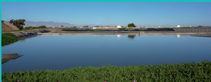
Agadir urban wastewater treatment – M'zar station – Secondary treatment (lagoon basin). February 2013. Photo taken by Lydia Herrmann. Creative Commons 2.0
