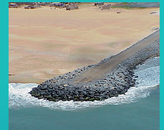
Groynes at the Keta Sea Defense Project on Ghana's coast. Kwasi Addo Appeaning Photo used with Creative Commons License.
