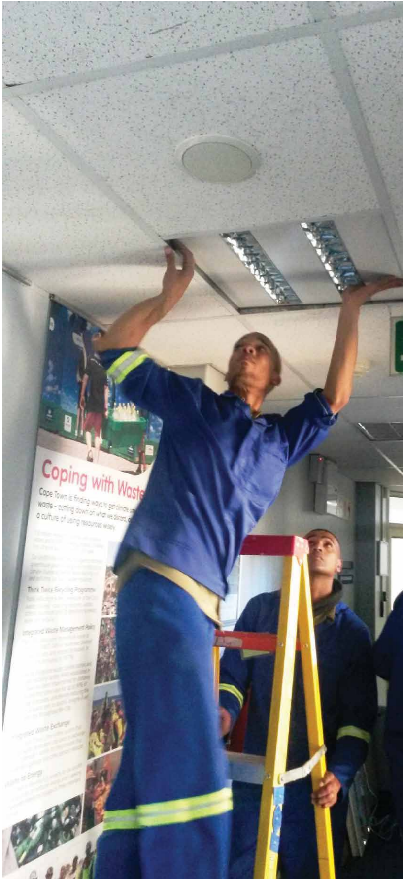
Energy efficiency retrofits in Cape Town Council operations in action.
