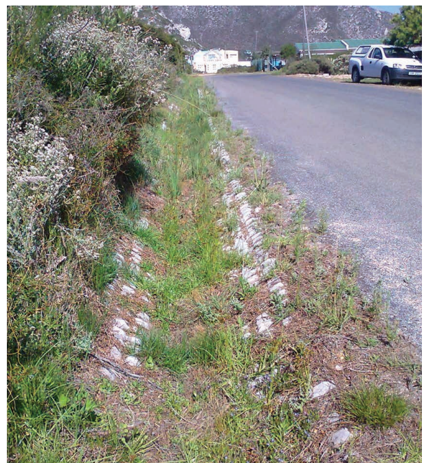
Figure 12: Bio-swale to enable stormwater filtration and infiltration (KZN)
