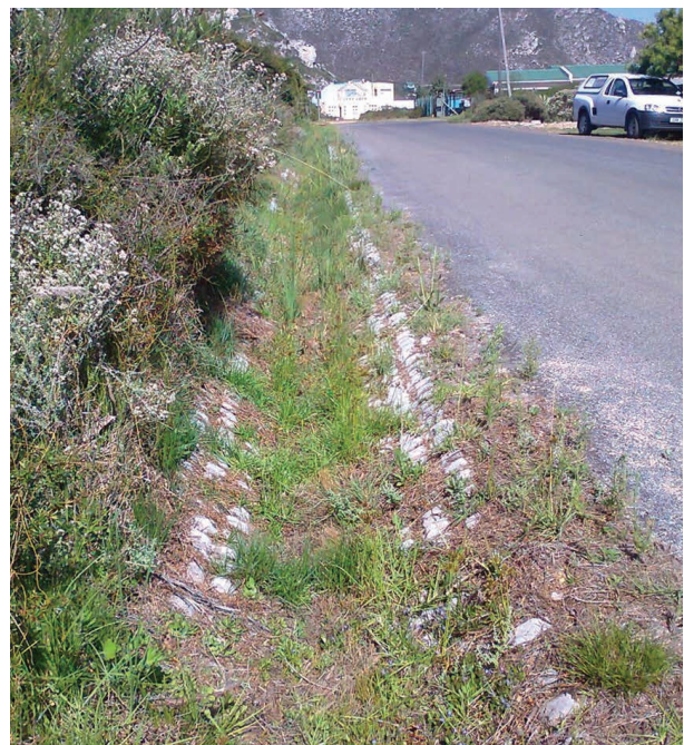
Figure 12: Bio-swale to enable stormwater filtration and infiltration
