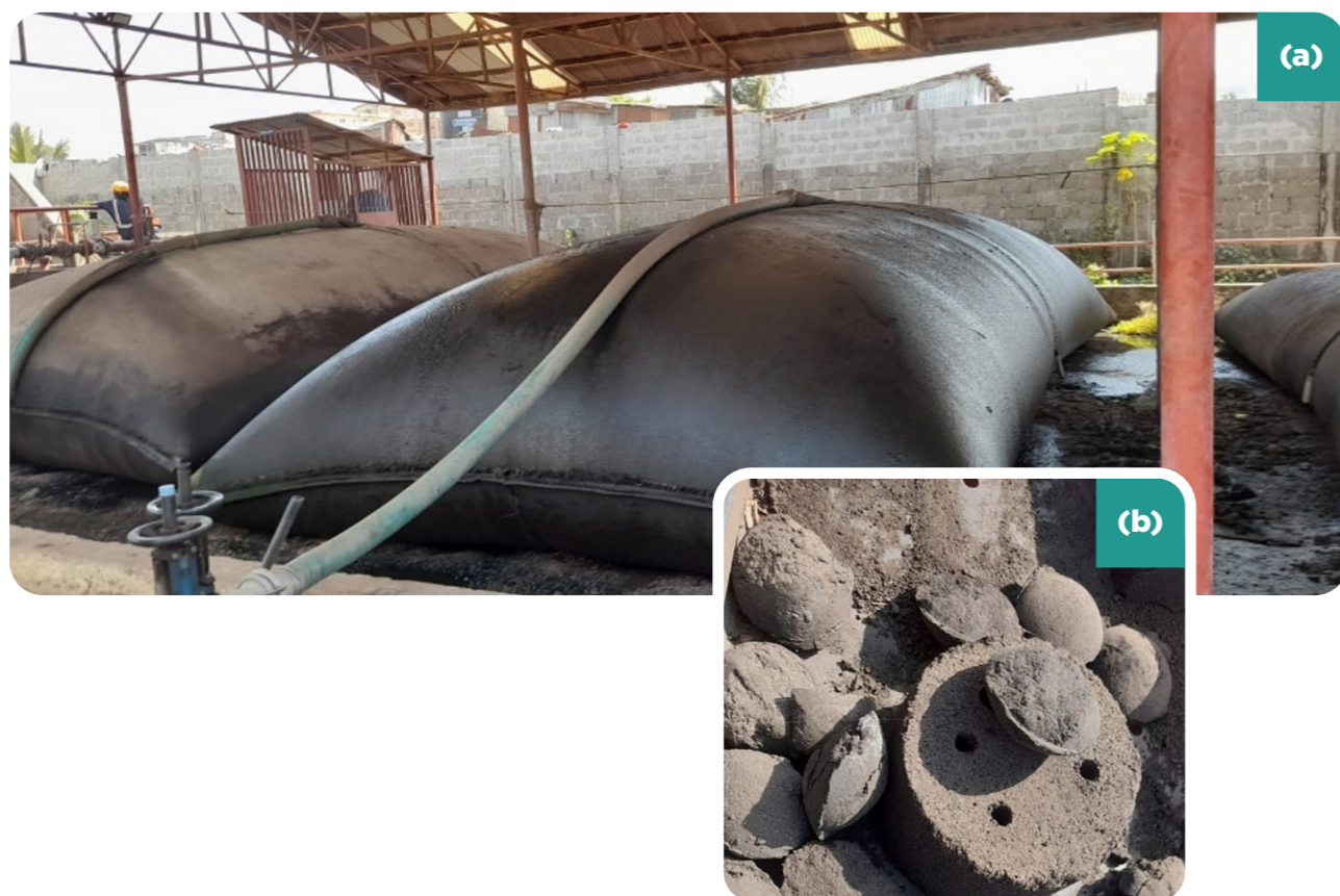
Figure 8: (a) Faecal sludge treatment facility managed by GOAL SL and (b) briquettes from treated sludge
