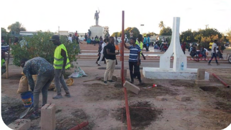
Figure 7: The site during the construction and greening work (Source: INTERACT-Bio team)
