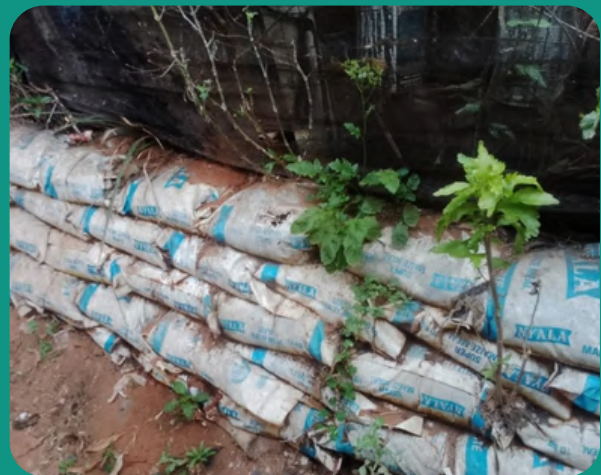
Residents of Pholani informal settlement in Durban are rebuilding after the 2022 floods, for example, we have decided using the sand bag strategy to close or fix the open places after the floods. Credit: INACCT Resilience
